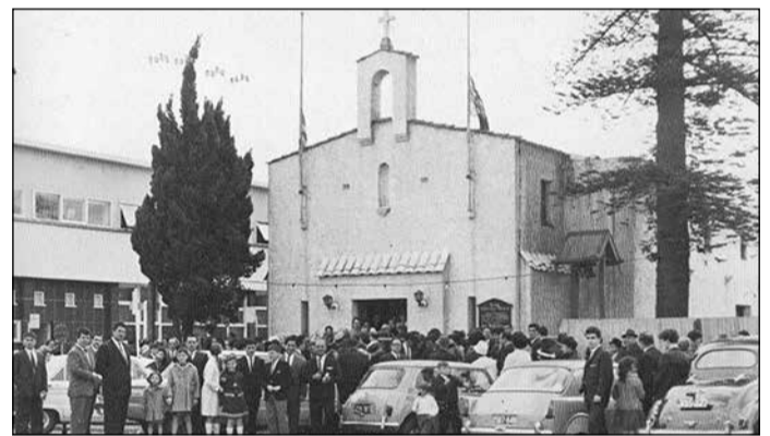
Franklin Street Cathedral. The first Greek Church in Adelaide
